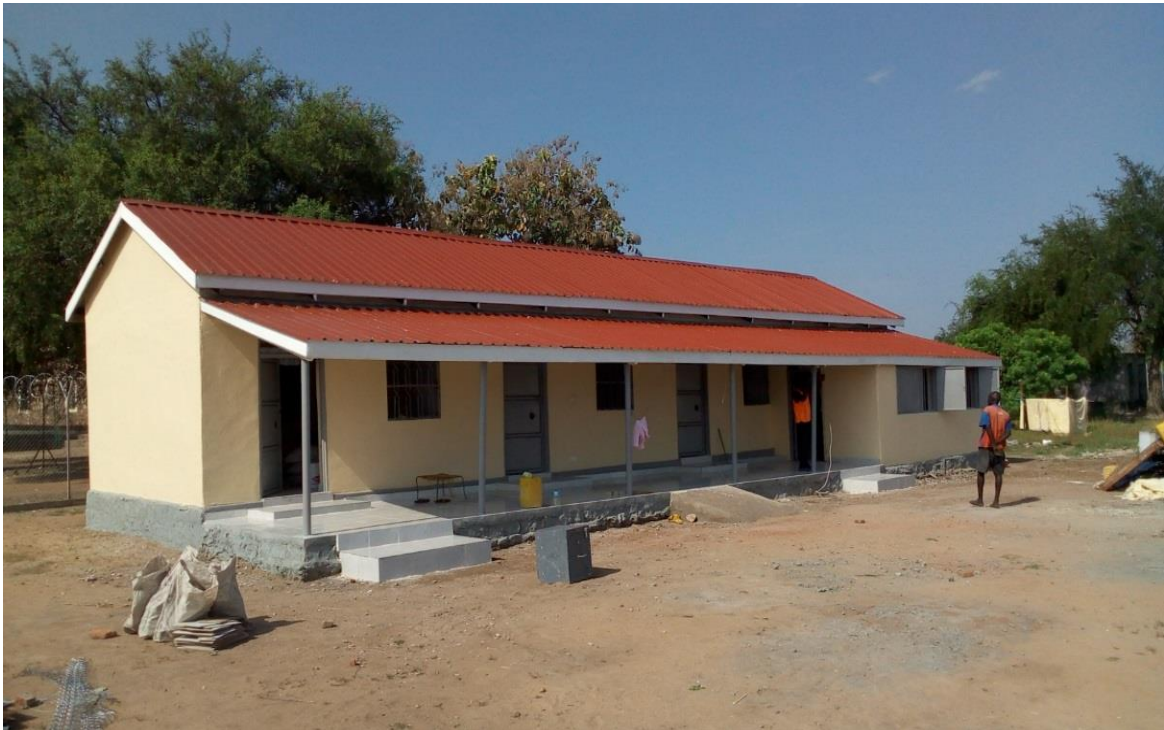
The County headquarters of Terekeka renovated in 2016
